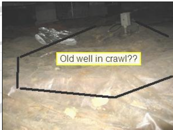
2.6 Picture 2 in crawlspace under new addition
