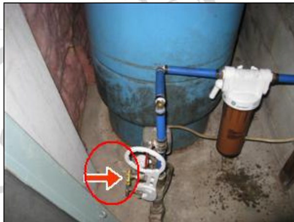
4.3 Picture 1 In basement
