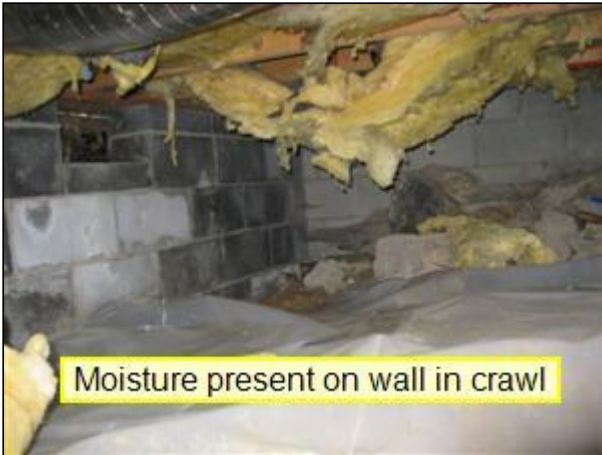
1.0 Picture 5 crawlspace under kitchen
