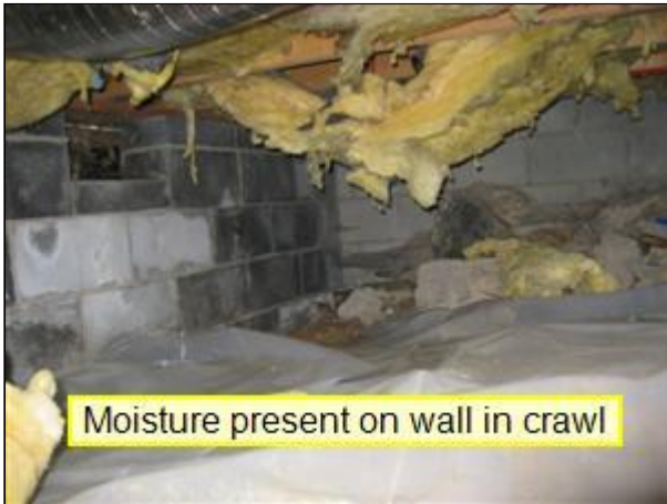
1.0 Picture 5 crawspace under kitchen
