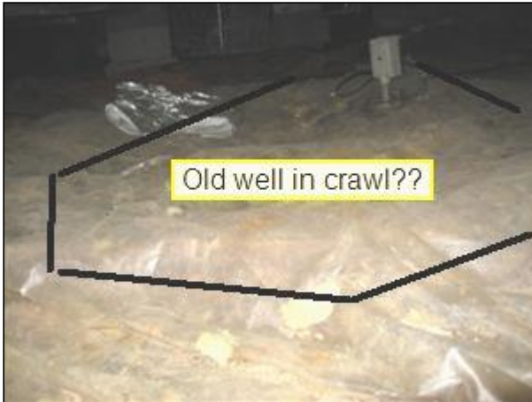
2.6 Picture 2 in crawlspace under new addition
